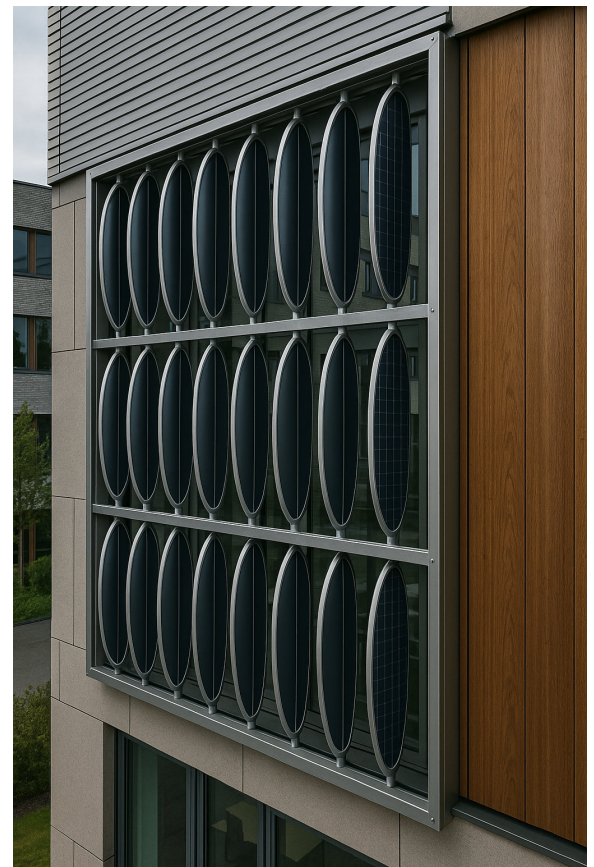
Figure 1: Schematic representation of PV-integrated shading
